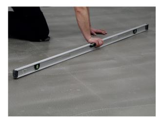
maximum 2 mm over a length of 20 cm. If the indicated deviation is exceeded, the subfloor must be evened out with a suitable filler or levelling compound, and a check must be carried out to determine if a sealer is needed.
