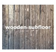
The glue down cannot be installed on most wooden substrates without special **preparation.** Either specific levelling compounds must be used, or the wood subfloor must be covered with special layers, e.g. plywood panels. These panels must be firmly attached to each other/the wood substrate and/or be glued or fixed. If there is moisture in the wood-based subfloor or there is no proper moisture barrier below the wood-based subfloor, it has to be removed first.
