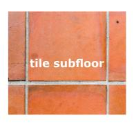
The glue down can only be installed on top of firmly levelled subfloor for all gaps between ceramic tiles will telegraph through. Installation directly on unlevelled top of ceramic tiles is not recommended!
