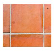
Check the subfloor for moisture problems. The joints of the new floor covering should never be aligned with the underlying tile joints. It is not necessary to fill the grouts of a subfloor comprised of ceramic tiles with joints when these do not exceed 5 mm in width. Bear in mind that some ceramic tiles may show rising edges/corners although the main level may be correct. These parts may telegraph through the floor covering in the future.
