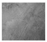
Let new concrete dry sufficiently. The moisture content of the subfloor must be less than 75% RH at min. 20°C. Max 2% CM for cement and 0.5% for anhydrite.
