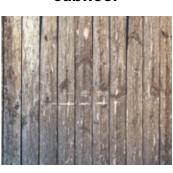
Check the floor for insect infestations. Make sure the subfloor is levelled and screw down any loose sections firmly. Wooden subfloors should always have access to air and should be ventilated at the edges.
