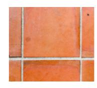
Zenn glue down can only be installed on top of a firmly levelled subfloor. All gaps between ceramic tiles will telegraph through. Installation directly on unlevelled top of ceramic tiles is not recommended!
